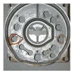
Flatten the tabs that hold the light tubes, bending them into the light holes. There are four dimples on the bottom near the Temp and Fuel gauge mounting holes that need to be flattened also.
